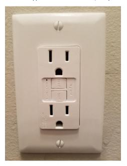
Each GFCI circuit has a TEST and RESET button. Once each month, press the TEST button. This will trip the circuit. To restore service, press the RESET button. If a GFCI breaker trips during normal use, it may indicate a faulty appliance and you will need to investigate the problem. One GFCI breaker can control up to two outlets.
