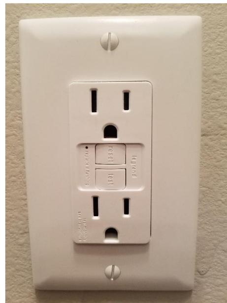
Each GFCI circuit has a TEST and RESET button. Once each month, press the TEST button. This will trip the circuit. To restore service, press the RESET button. If a GFCI breaker trips during normal use, it may indicate a faulty appliance and you will need to investigate the problem. One GFCI breaker can control up to two outlets.
